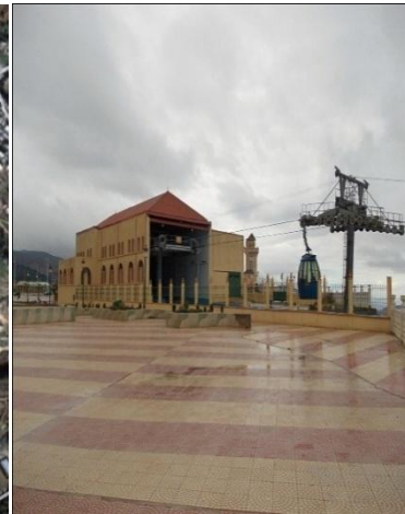
Fig.4. Cable car lift to the plateau
